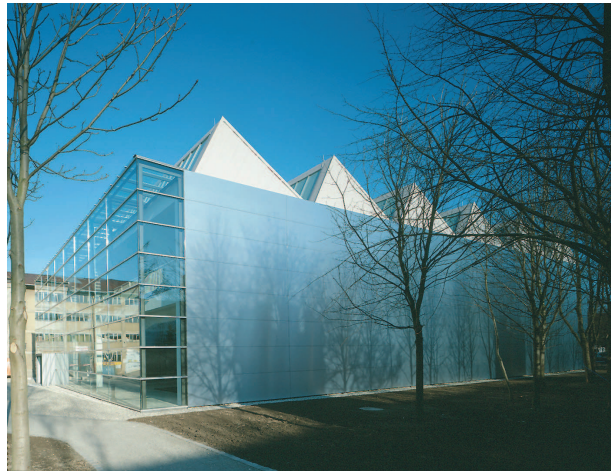
Figure 22: Alf Lechner Museum, Ingolstadt (southwest side) The rear-ventilated cladding has a gap of 25 cm to the outside wall.
