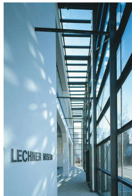
Figure 24: Alf Lechner Museum, Ingolstadt (inside view of the glass façade looking southwest). The gap between the glass façade and the preexisting structure forms a 10 m high shaft that is without hot-air currents in the heating season.
