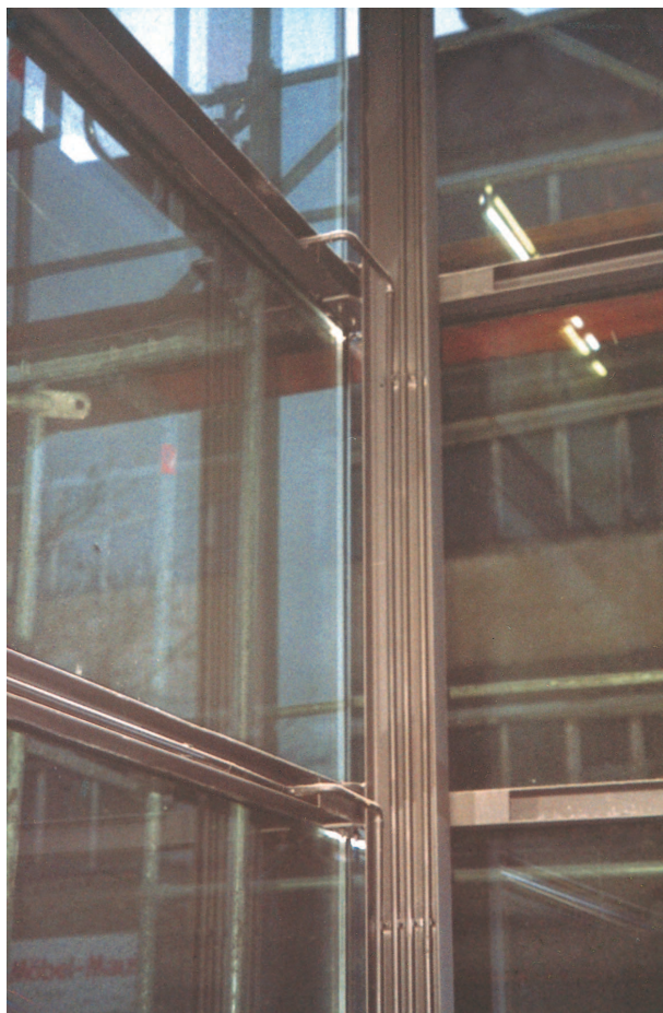
Figure 28: Alf Lechner Museum, Ingolstadt, Northeast Corner of Glass Façade , from inside. In the corner post are the feed lines to the two tube loops of the façade ( \varnothing = 18 \text{ mm} ) at the heights of the floors (ground floor: 3rd and 4th horizontal steel U-beams, upper floor: 6th and 7th horizontal steel U-beams of the framework for supporting the glass. All tubes are painted and held in place by plastic clips. Left: ground floor loop foreline (in lower U-beam) and return line (in upper U-beam).
