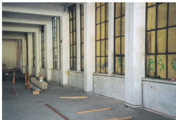
Figure 29: Alf Lechner Museum, Ingolstadt, Ground Floor. Southwest wall, with wall-base and windowsill-height heating tubes ( \varnothing = 18 \text{ mm} ), before the window niches were plastered and the concrete "baseboards" were poured.
